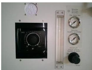
Figure 77 Control panel with the diaphragm pump
